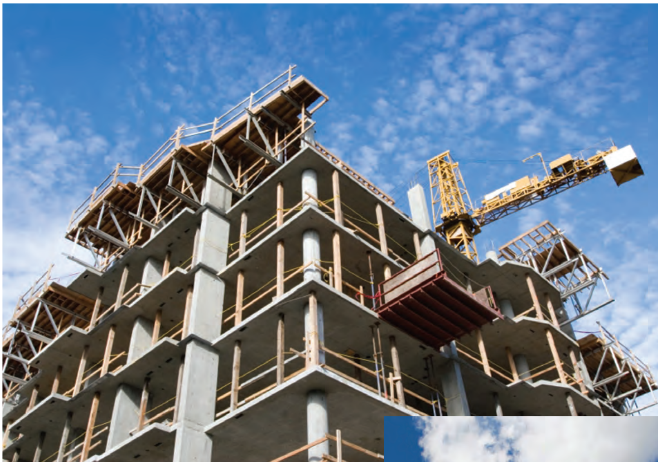
Construction Elevator Emergency Stops
