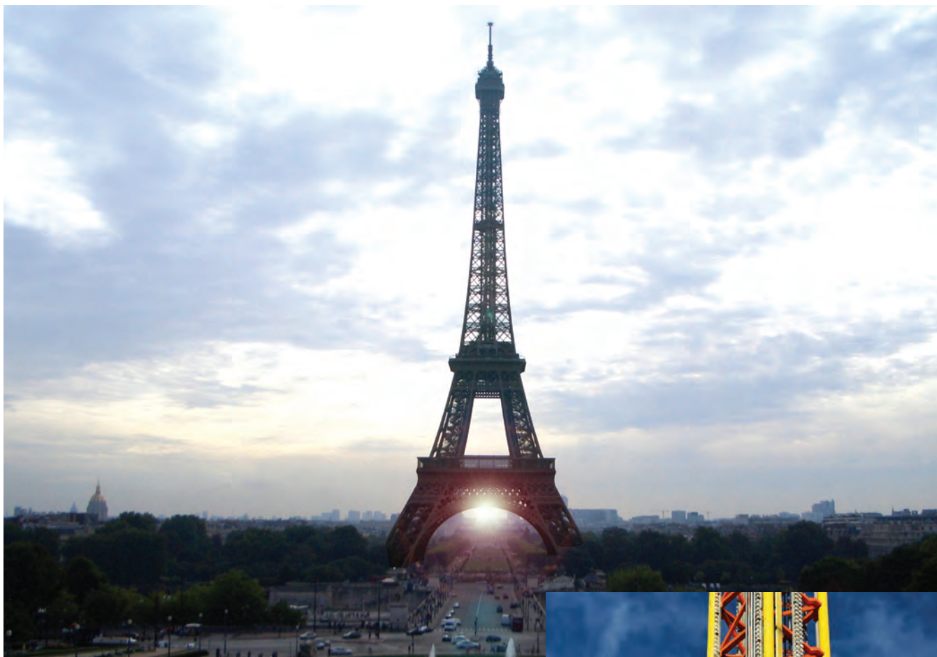
High Speed Elevator Applications
